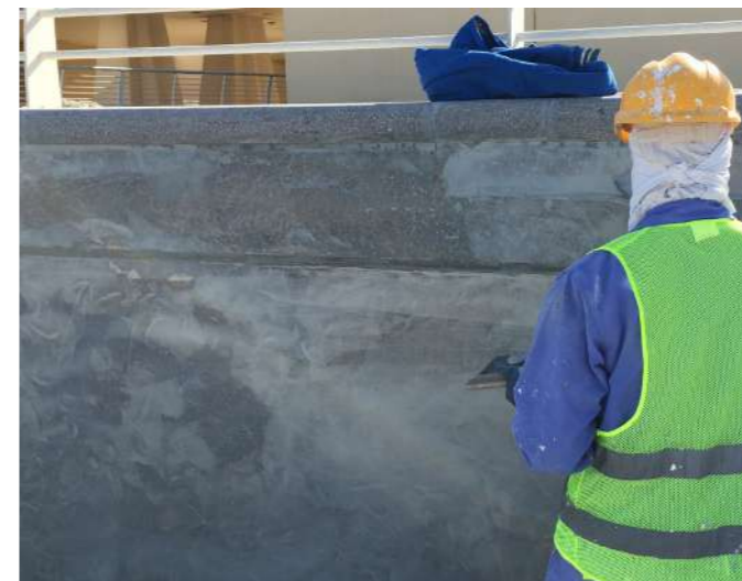
Small scale face filling between coats
