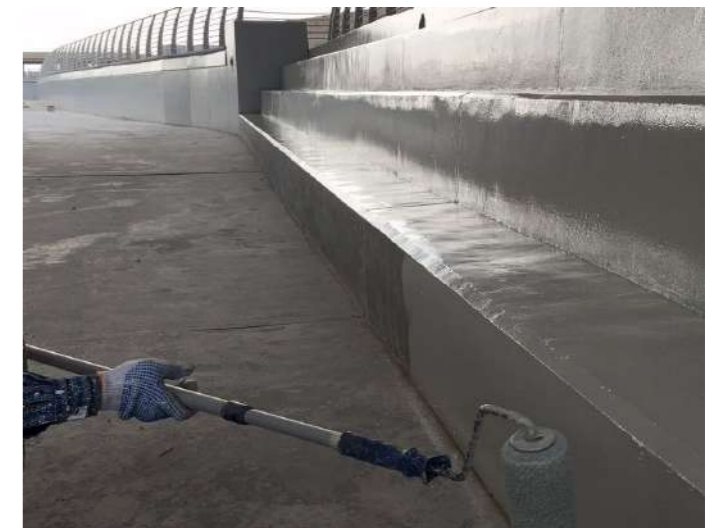
Apply the protective coating system
