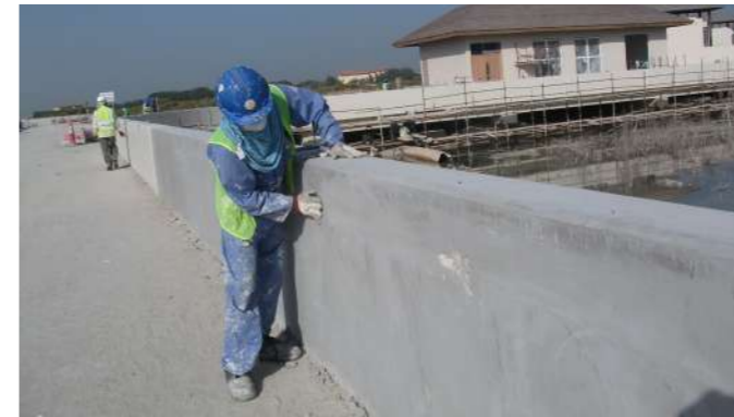
Prepare and repair
