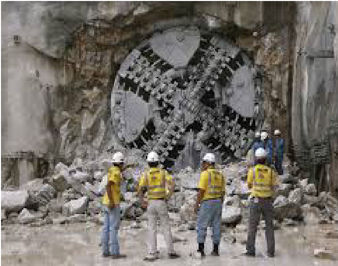
TUNNEL BORING MACHINE
