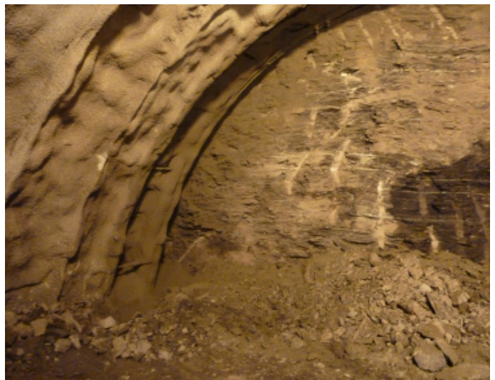
DRILL & BLAST METHOD
