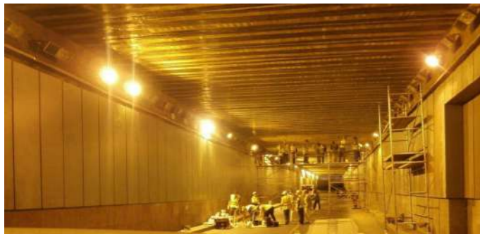
Nitoplate installed in night shifts using temporary access scaffolds
